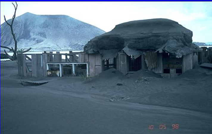
Roof collapse
