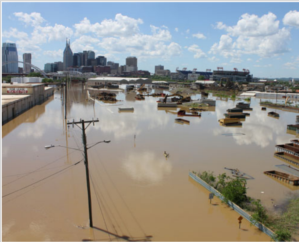
Figure 4: Flood damage in Nashville, TN from heavy rainfall on May 1–2, 2010 Parts of Middle Tennessee received more than 19 inches (49 cm) of rainfall in two days. Floods this severe are expected only once per 1000 years but may become more commonplace in a warmer world.
