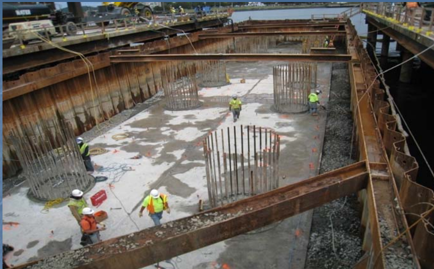
Marine enclosure dry with shafts ready for construction at Tower Pier 2
