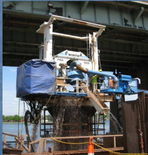
Pile-top reverse circulation drill
