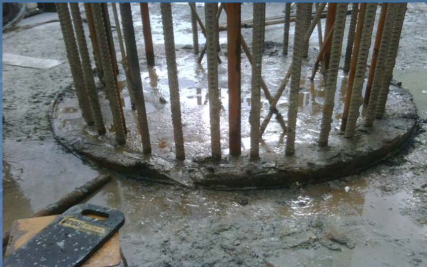
Drilled shaft after marine enclosure pumped dry
