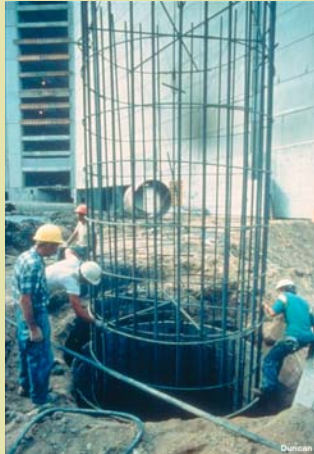
Placing the Rebar Cage
