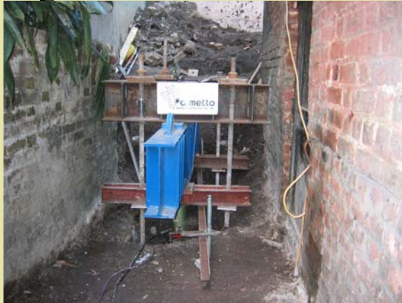
Static Load Test 50 Broad St., Charleston, SC
