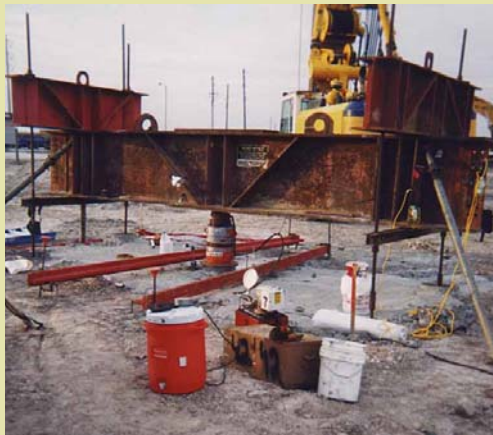
Static Load Test on DD Pile Photograph courtesy of WPC Inc.
