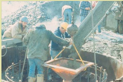
Placing Concrete using Tremie
