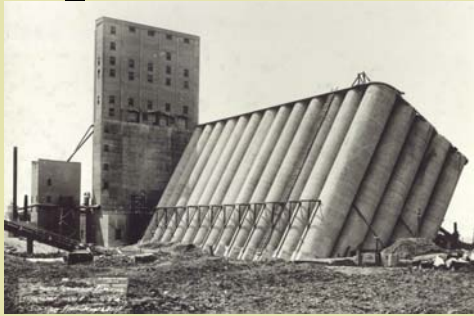
Transcona Grain Elevator Winnipeg, Manitoba October 18, 1913 Tilt: 27°
