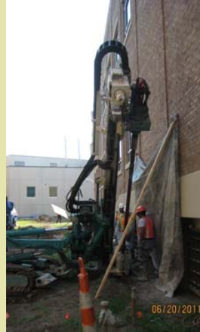
Micropile Seismic Retrofit (Photograph courtesy of Palmetto Gunite)
