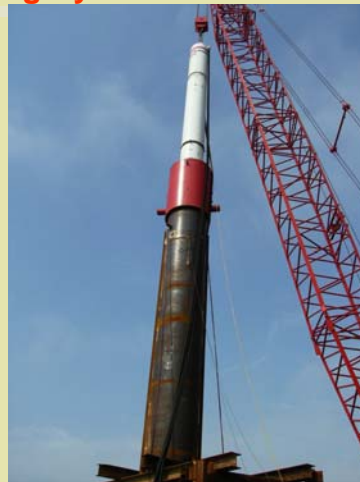
IHC S-600 Hydraulic Hammer: Rated Energy ~440kip-ft (600kN-m)
