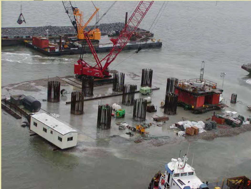
West Tower – Arthur Ravenel Jr. Bridge
