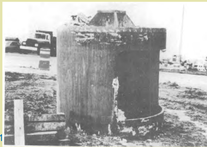
Figure 4.6 A typical “muck bucket” or “clean-out bucket” (O'Neill & Reese, 1999)
