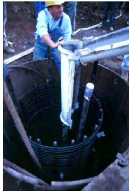
Figure 9-1. Free Fall Concrete Placement in a Dry Excavation (FHWA NHI-10-016).
