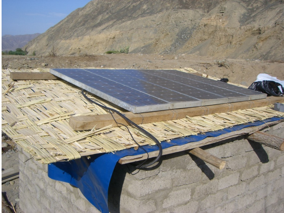
Figure III-16 PV installation in Turripampa
