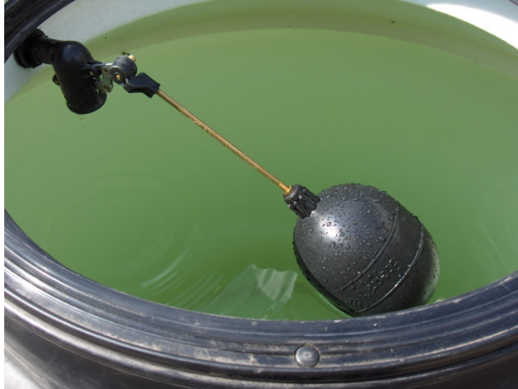
Figure III-15 Tank float valve
