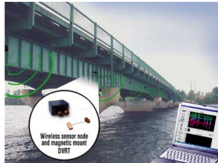
3. Wireless sensors are used to measure long-term stress and strain in civil engineering structures like buildings and bridges. (Courtesy: Microstrain Inc.)
