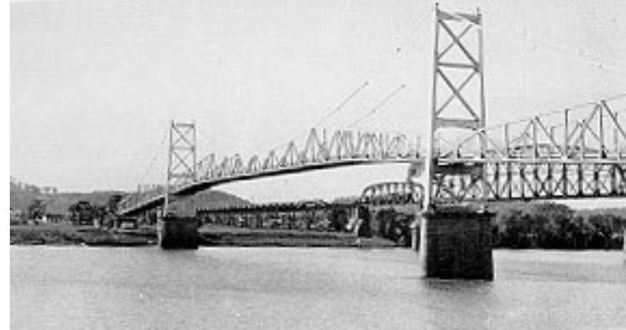
The Silver Bridge connecting Point Pleasant, West Virginia, over the Ohio River, U.S.A.
