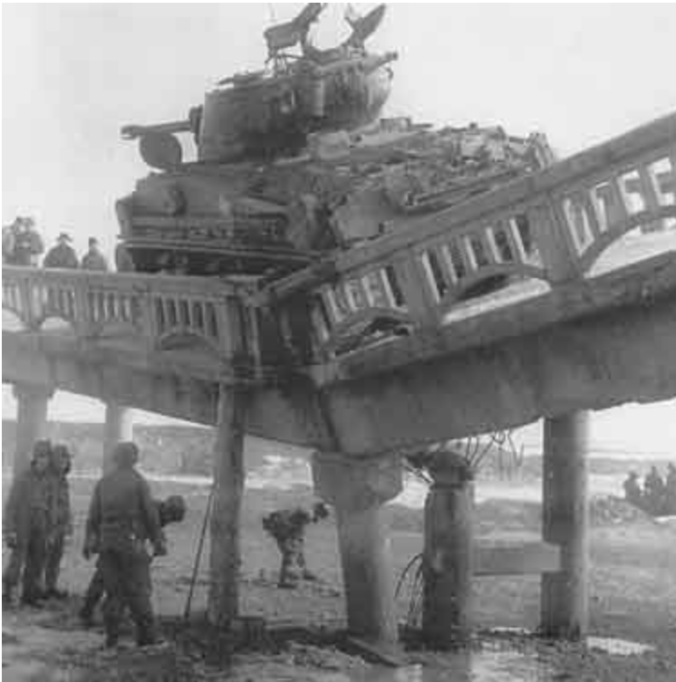
Pedestrian bridge failed due to overloading by a tank
