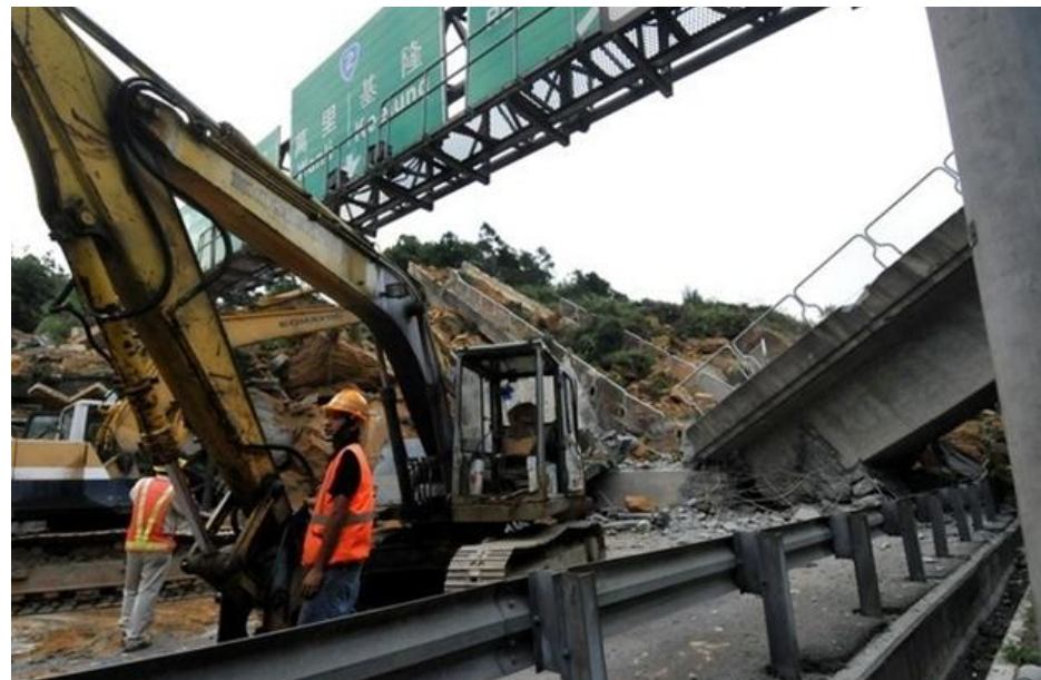
2010 Chi-du landslide, Taiwan
