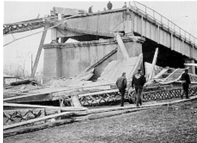
On December 15, 1967, the Silver Bridge collapsed while it was full of rush-hour traffic, resulting in the deaths of 46 people.
