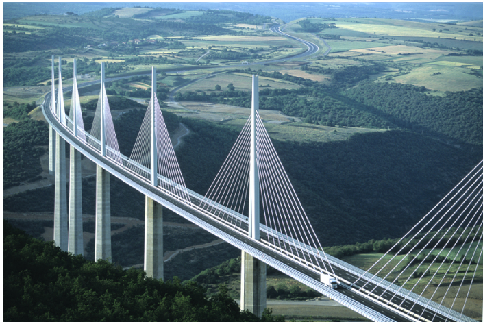
Millau Viaduct Bridge, France (2,460 m)
