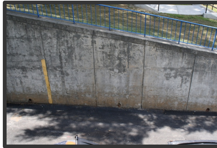
Fig 45: (left) Olney auditorium Fig 46: (Center) Olney receiving dock Fig 47: (right) Pinanski hall
