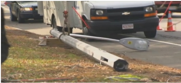
Fallen light pole in Massachusetts
