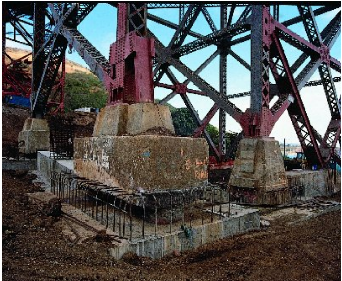
Foundation of the Golden Gate Bridge, CA
