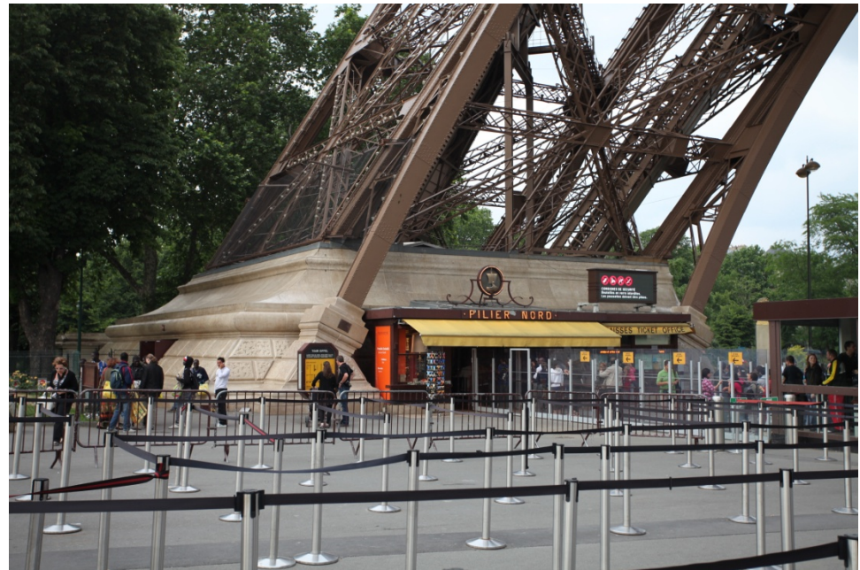
Northeast support of Eiffel tower, Paris, France
