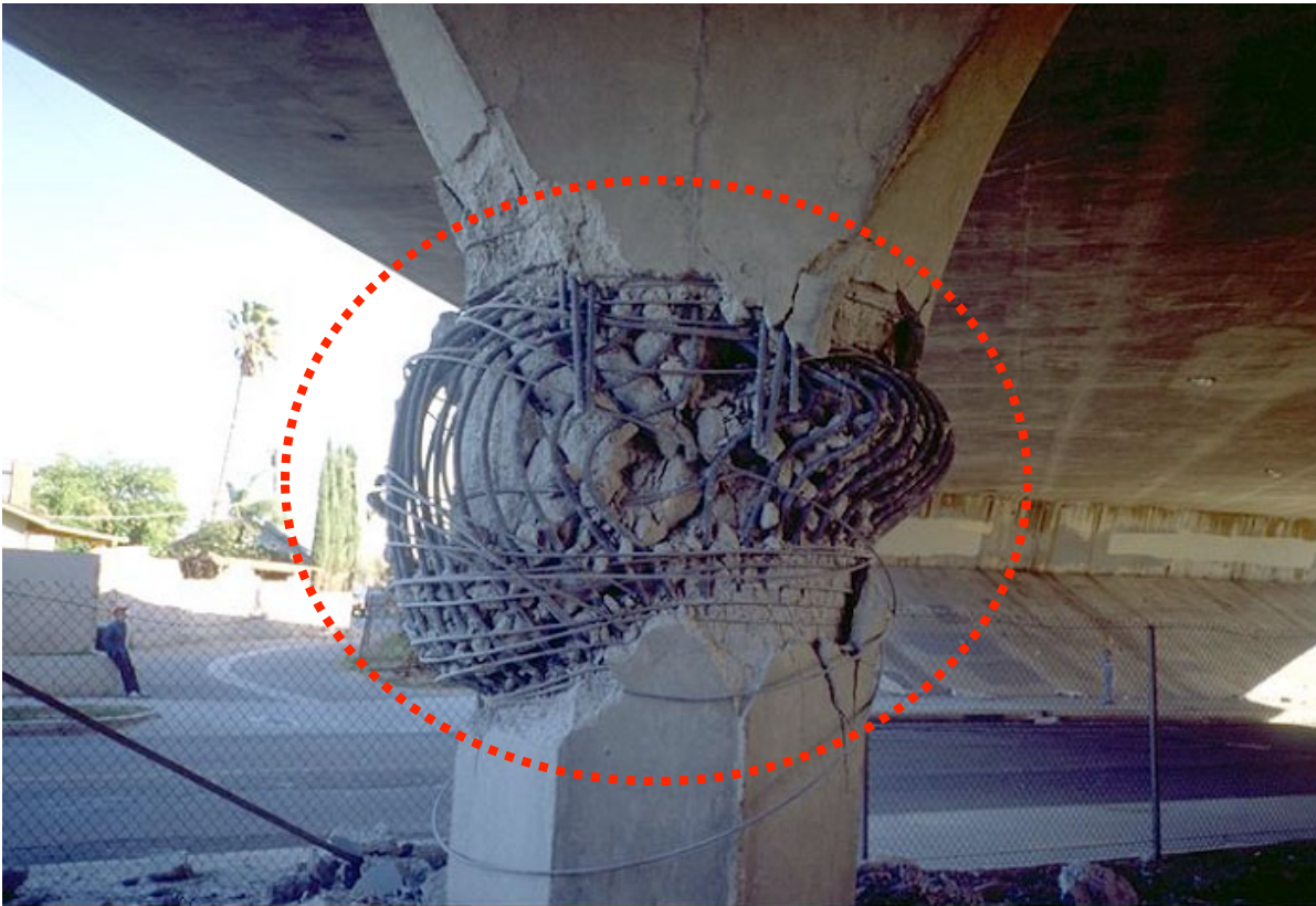
Buckling of a reinforced concrete bridge column
