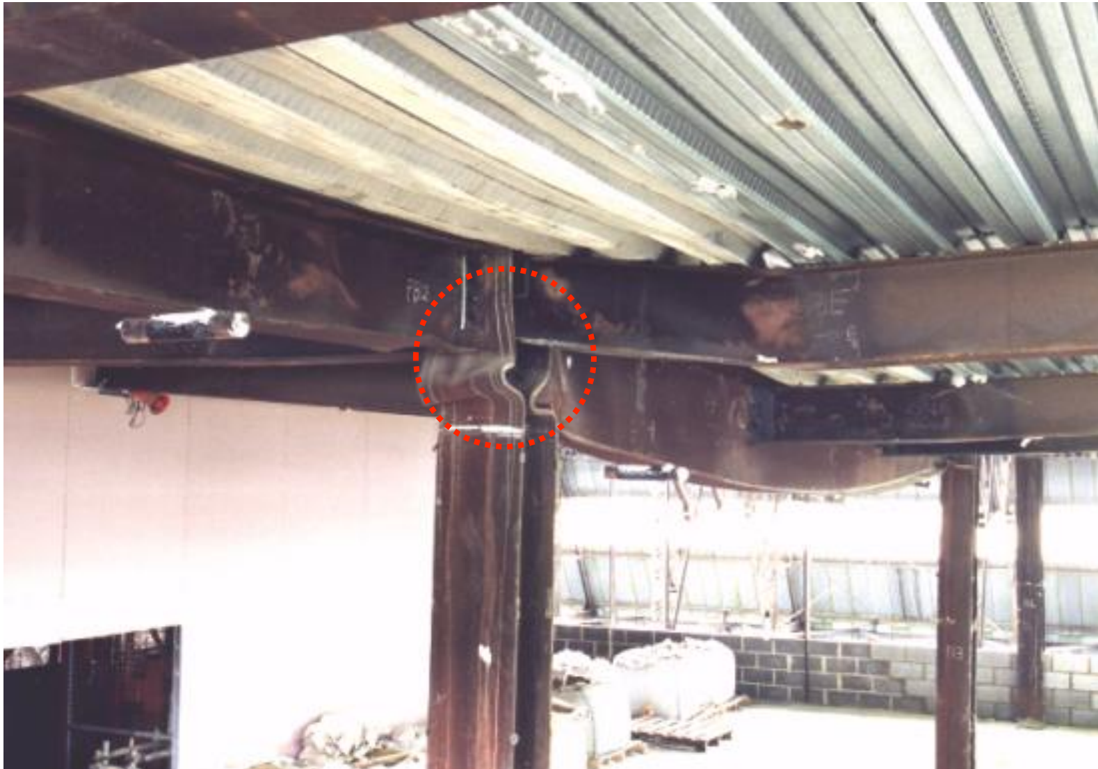
Buckling of a steel column
