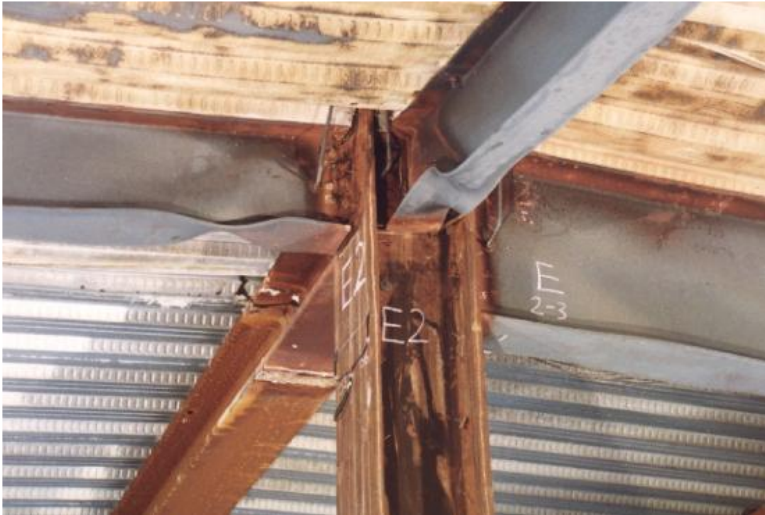
Buckling of a steel beam-column
