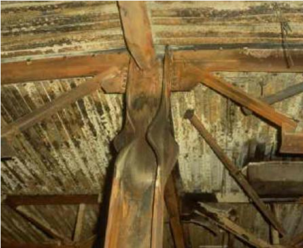
Torsional buckling of an I-beam members (Source: The Steel Construction Institute )
