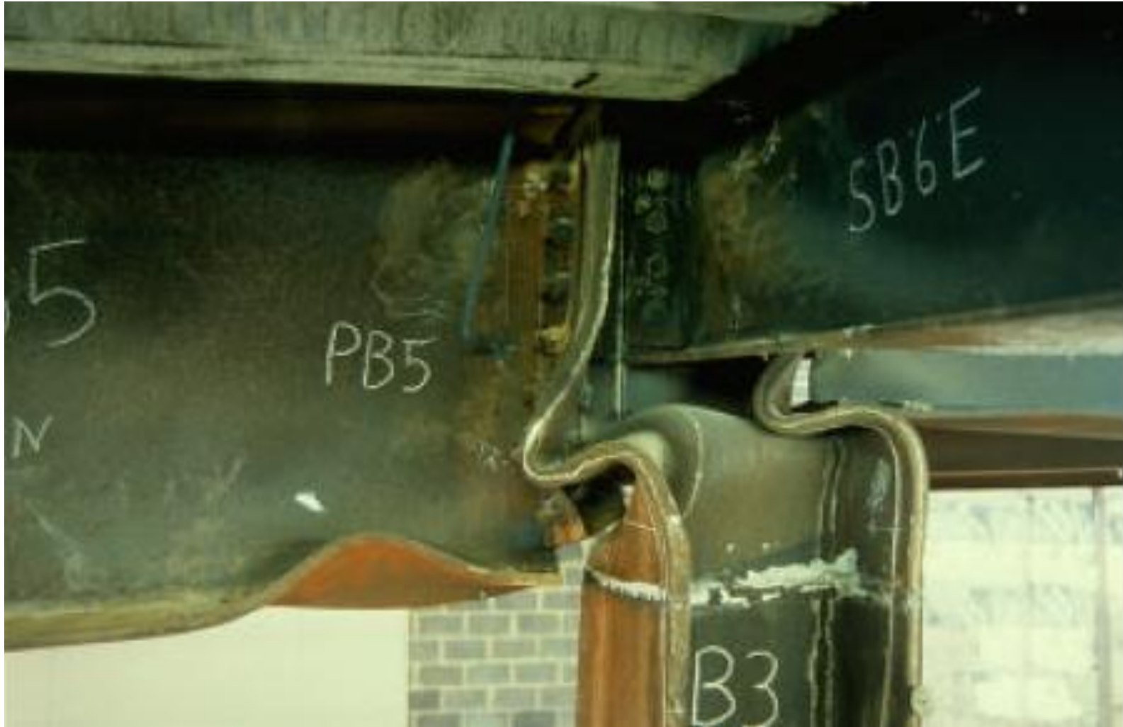
Torsional buckling of I-beam members (Source: The Steel Construction Institute )
