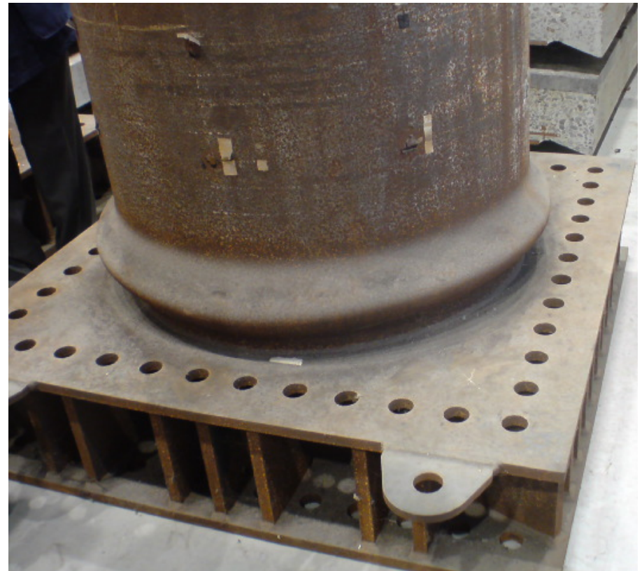
Local yielding at the bottom of a steel column, Public Works Research Institute (PWRI), Tsukuba, Japan (Source: T. Yu)
