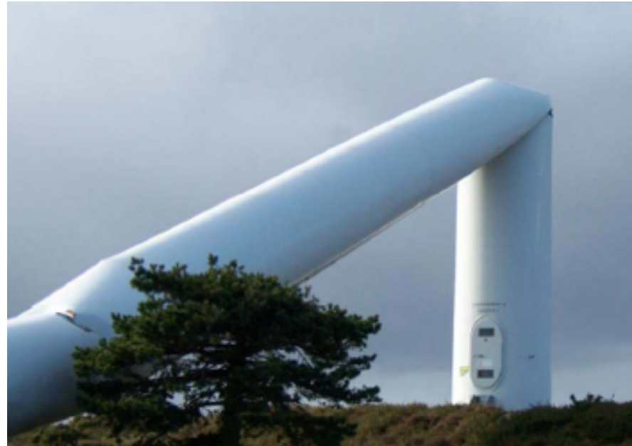
Failure of a wind turbine tower (Source: Greenward Technologies, Inc.)
