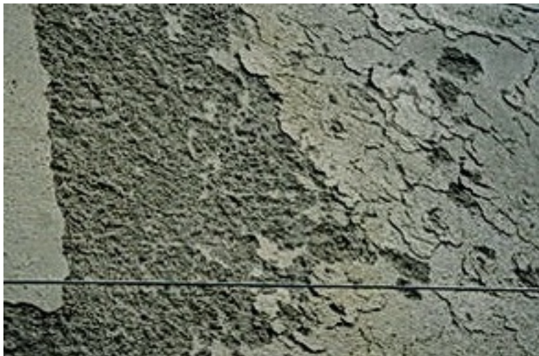
Figure 4.1 Concrete Segregation
