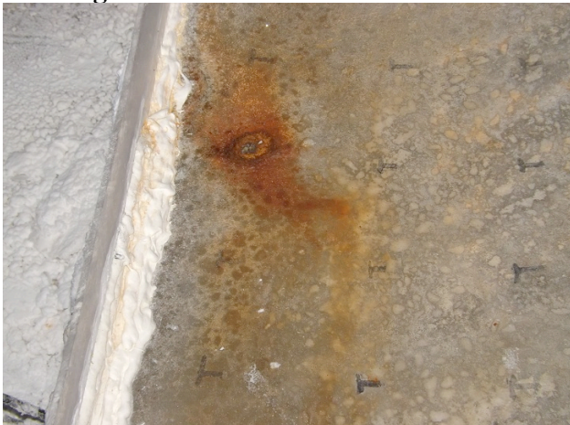
Fig. 5 Close-up surface rust location on the left of slab 1
