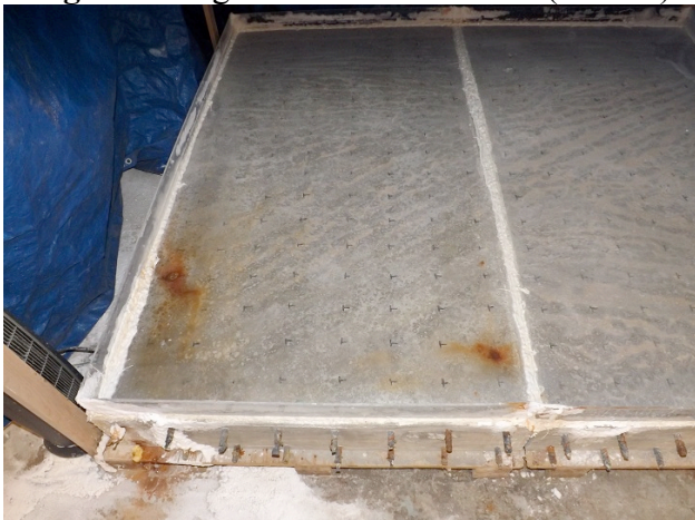
Fig. 4 Surface rust locations on slab 1
