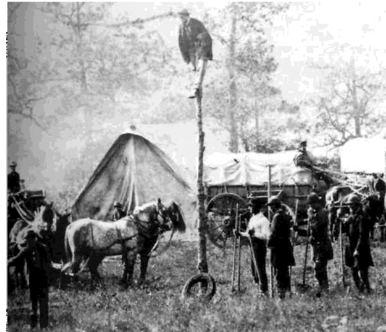
Telephone Line Installation Crew
