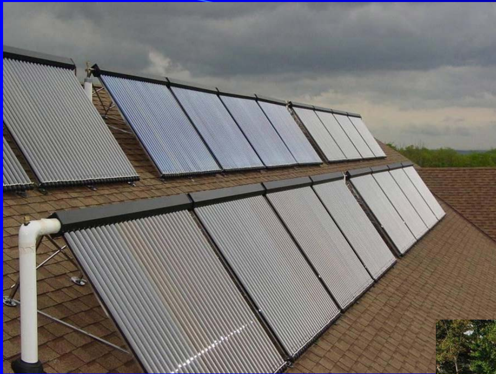
Active solar heating
