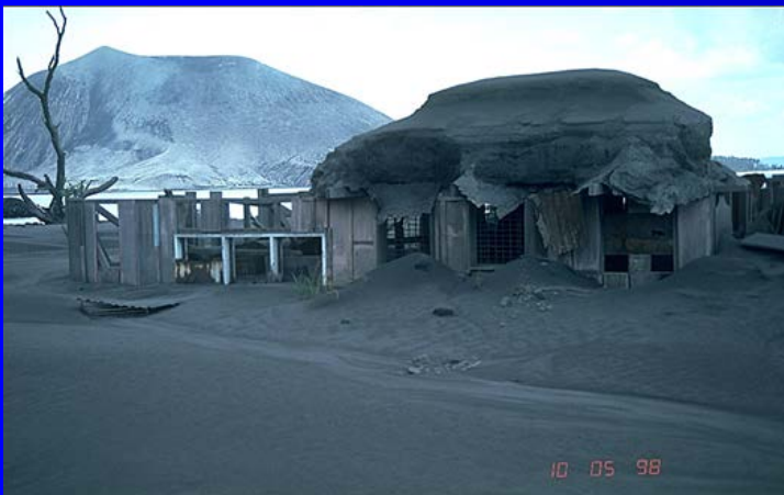
Roof collapse
