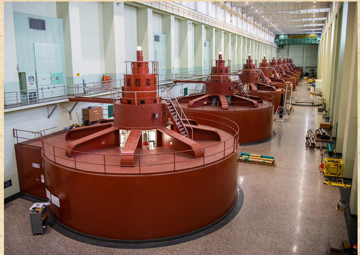
Grand Coulee Dam – Left Power House
