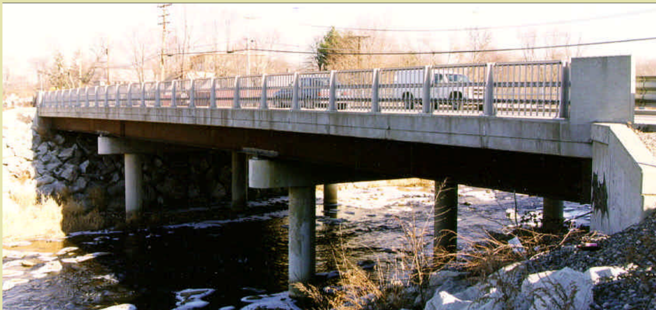
Bridge #9, Fitchburg MA
