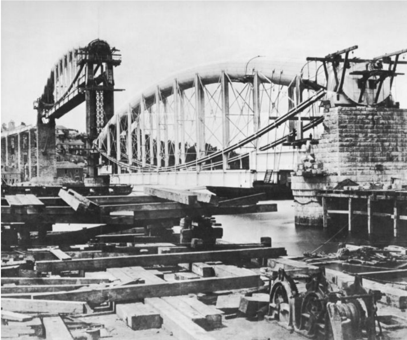
Royal Albert Bridge, UK (1859)
