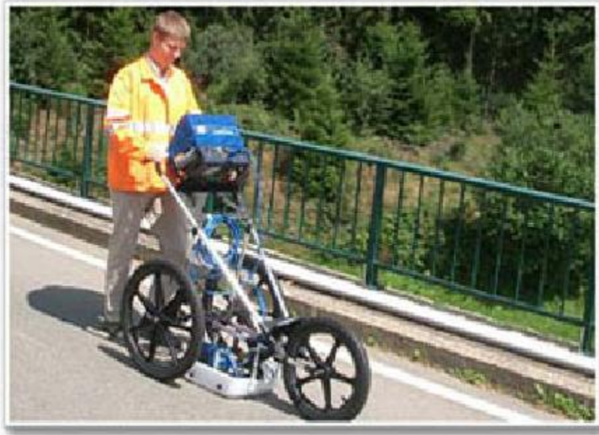
Figure 1-1: Bridge deck evaluation using GPR [ source : GSSI ]
