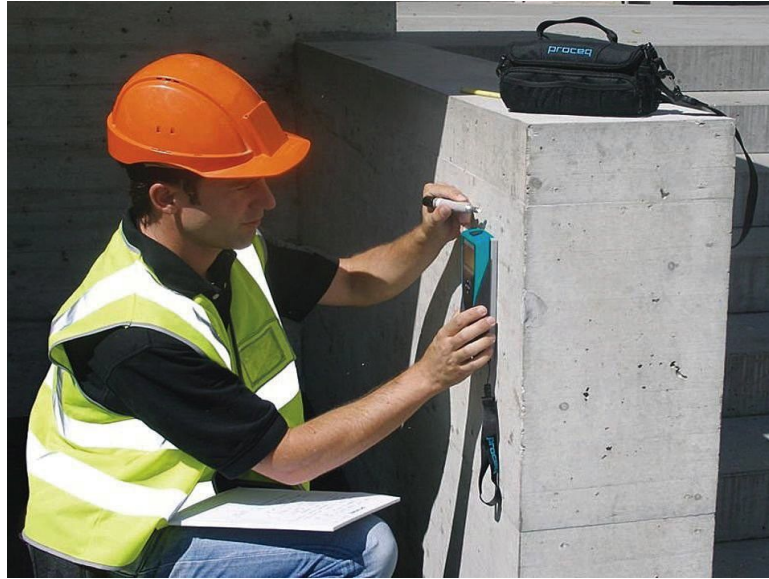
Figure 2-6: Field Inspection Using Covermeter [Source: Proceq®]
