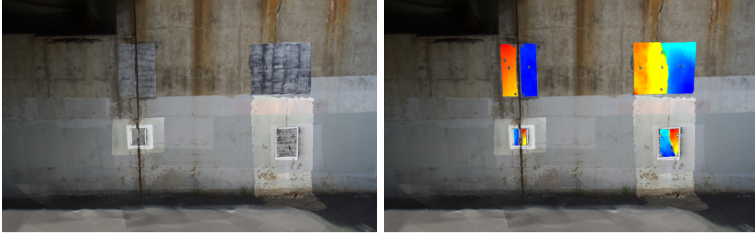
Figure 5-6: DIC integration at Lincoln Street bridge, Lowell MA.
