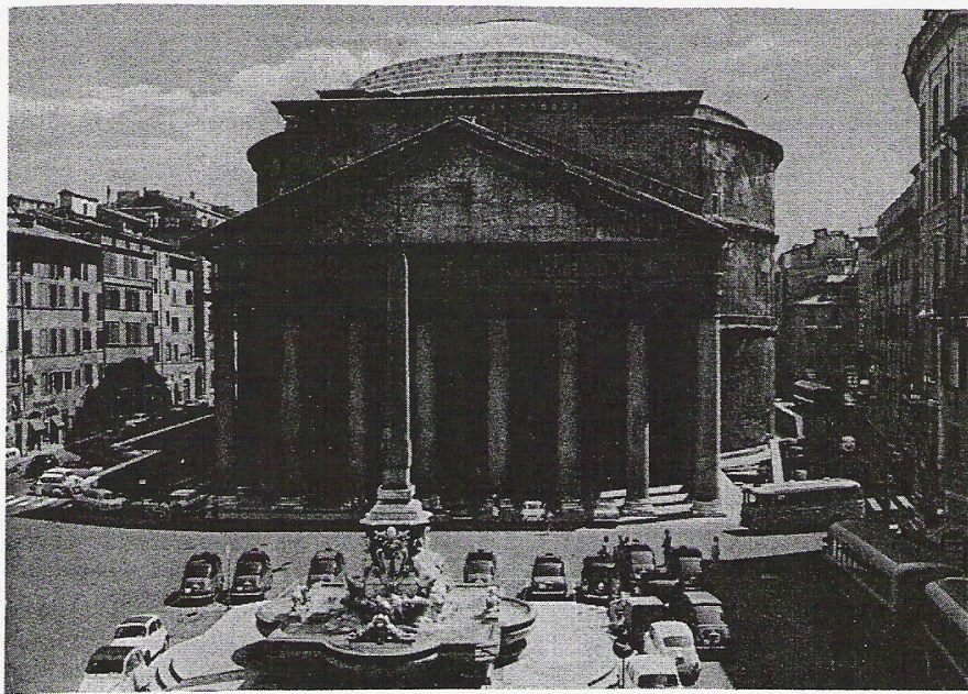
Fig. 1-3 (a) Pantheon, Rome, Italy, Dome Span = 43.4 m; Dome Rise = 21.6 m
