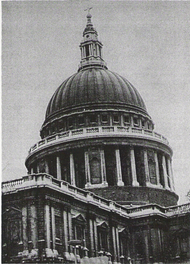
Fig. 1-8 St. Paul's, London, England, Dome Span = 30.8 m; Dome Rise = 33.5 m
