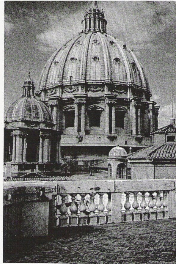
Fig. 1-7 St. Peter's, Rome, Italy. Dome Span = 41.6 m; Dome Rise = 35.1 m
