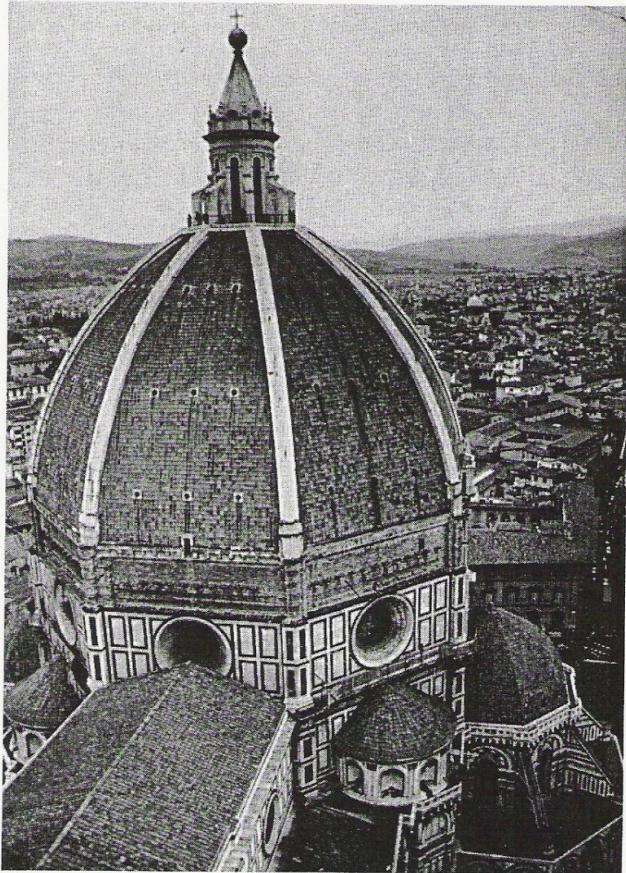
Fig. 1-6(a) S. Maria Del Fiore, Florence, Italy. Dome Span = 42.4 m; Dome Rise = 36.6 m
